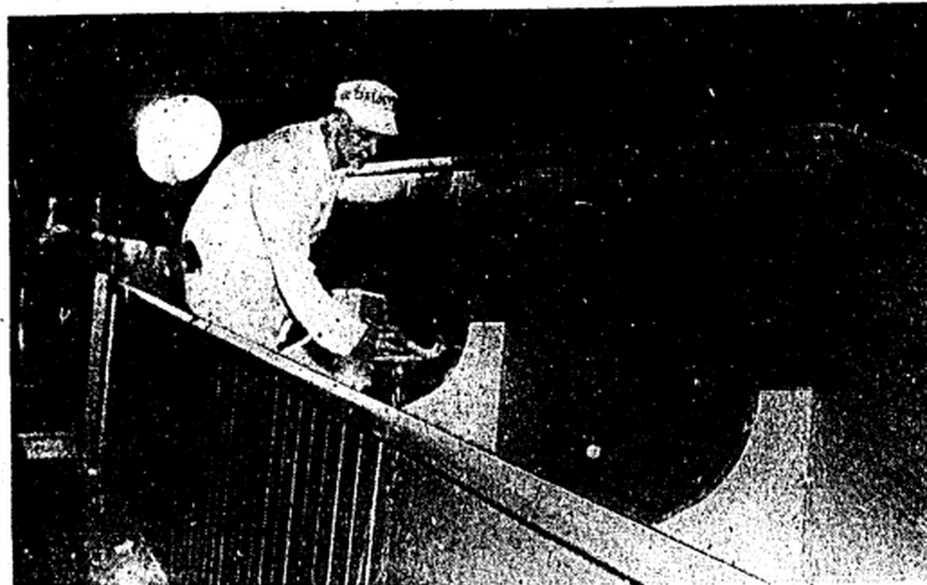
Dave Laskey Adds Coat of Paint to New Seats in Grey Section of Maple Leaf Gardens Workmen are adding 18 seats to each corner. Fifty will be ready for tonight's playoff game.
